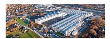
ALVANCE ALUMINIUM DUFFEL BV, a company of GFG Alliance, has an integrated aluminium plant, situated in Duffel, Belgium, equipped with casters, mainly used for internal scrap remelting, a hot rolling mill, three cold rolling mills and a large number of finishing and conditioning lines.
