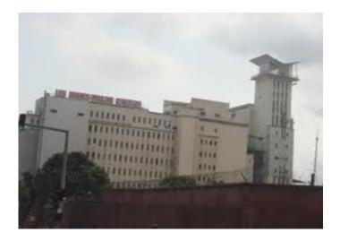
The silos of the Big Moulins of Abidjan (GMA) have been constructed in the 1960. Wheat, rye and other ingredients necessary to manufacture bread were stored there. The capacity of the silos is about 30.000 tons.
